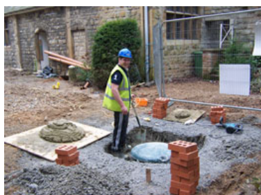
Rainwater harvesting tank being sunk
